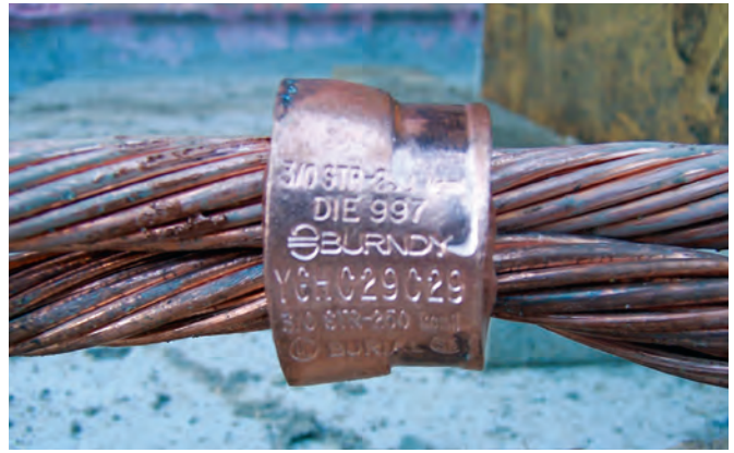
Figure 15. Properly crimped cable connection
