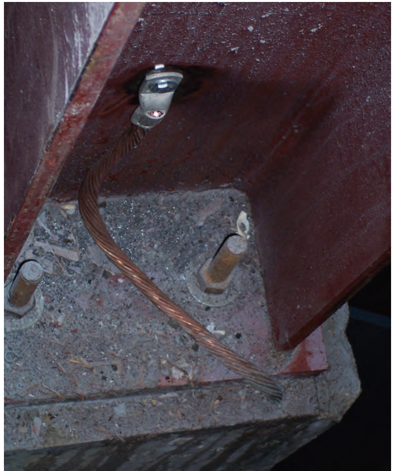
Figure 10. Proper ground connection to wall support
