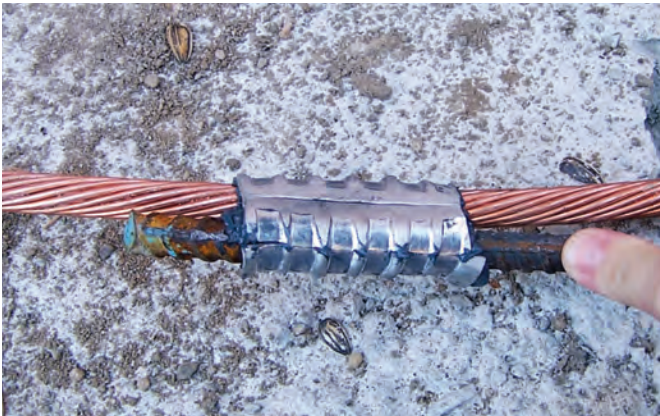
Figure 14. Properly crimped cable connection
