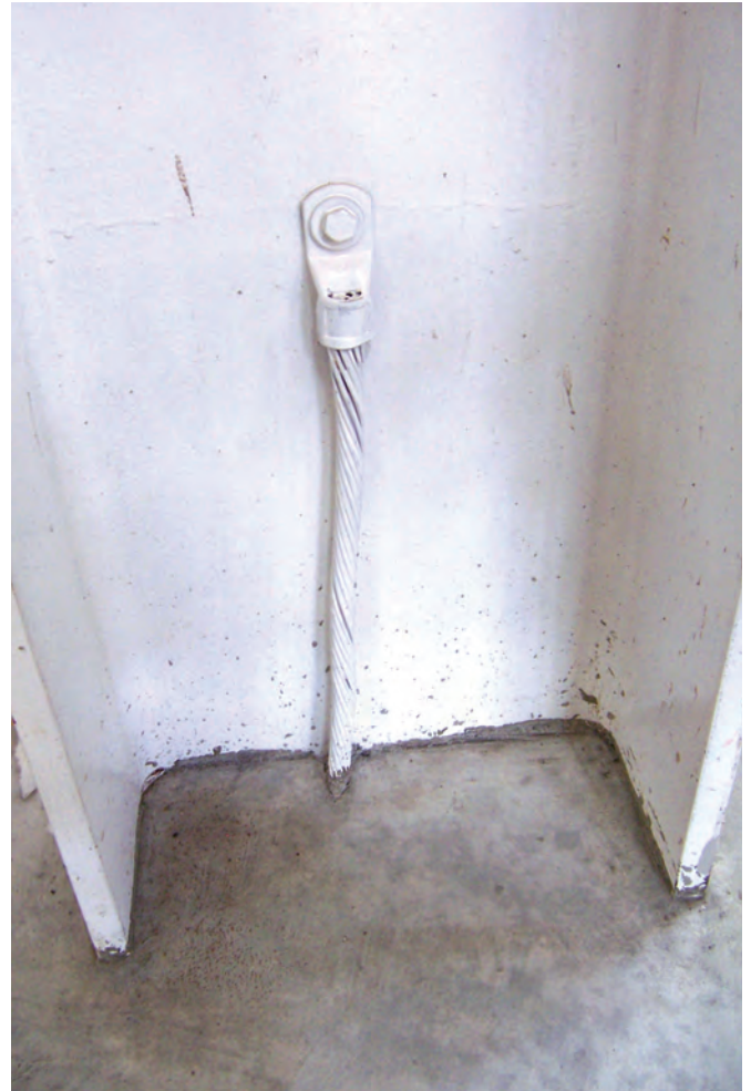
Figure 3. Ground connection made to metal beam before painting
